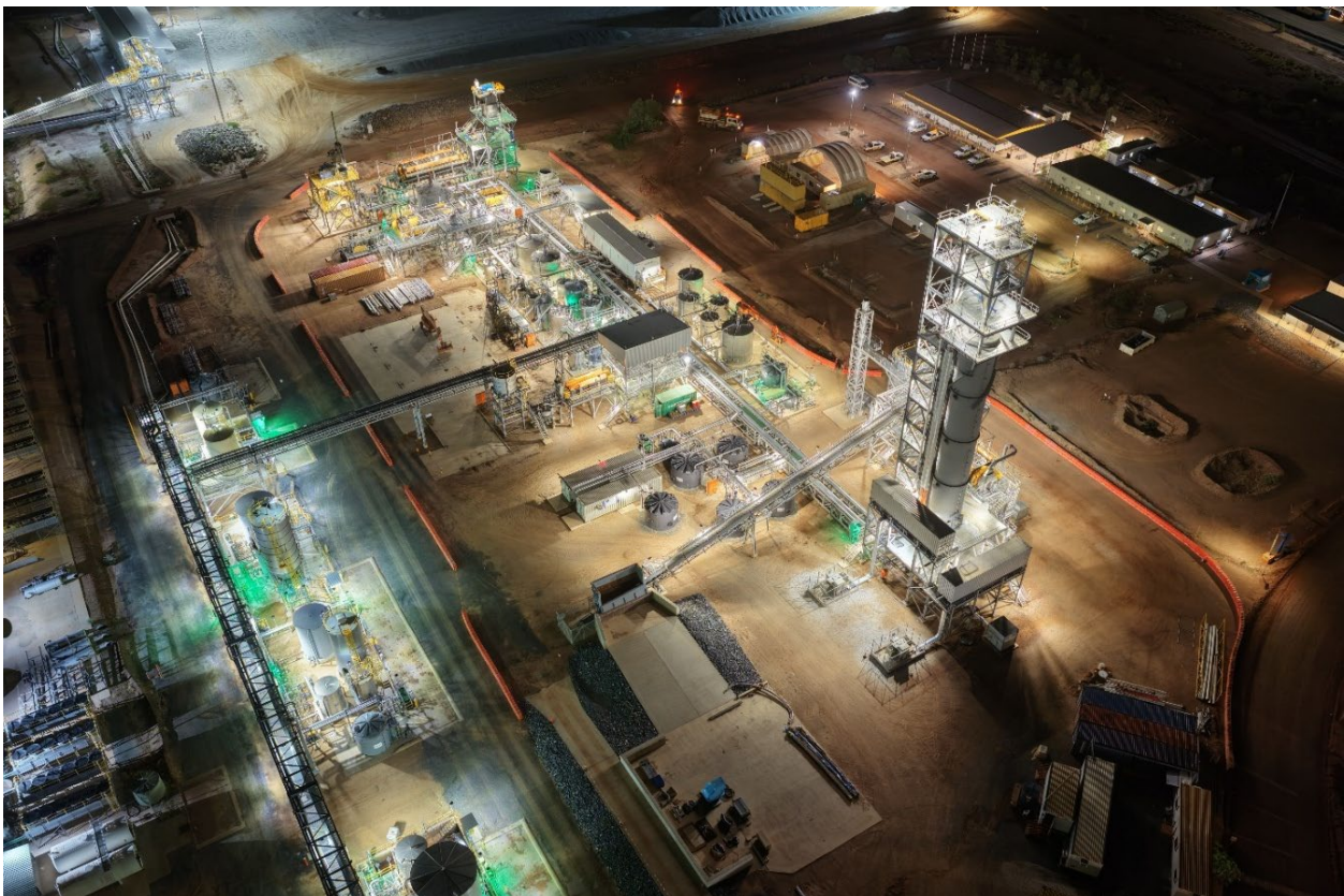
Figure 1: Mid-Stream Demonstration plant as at 2 April 2026.
