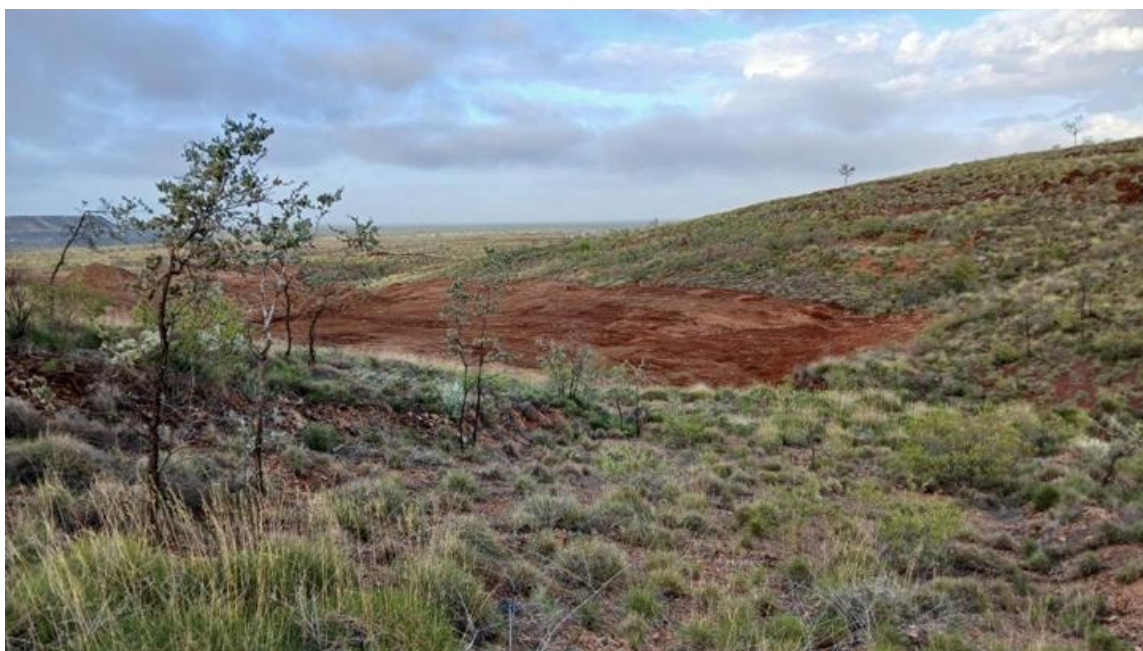
Plate 1 Lynas Find Haul Road clearing
